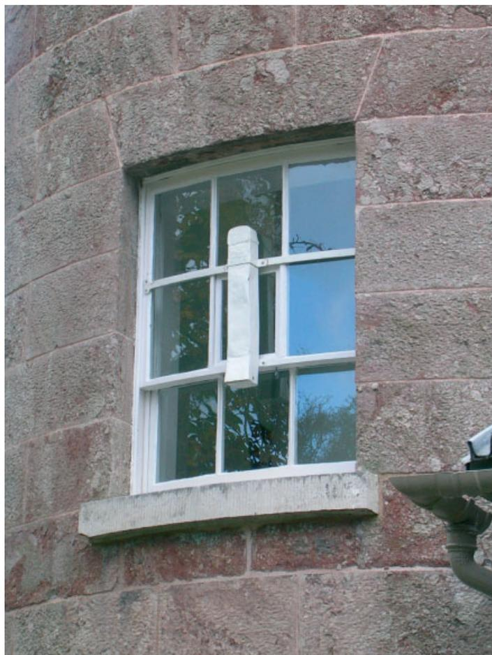
Figure 4. The light metal box at the north window of the East Tower at Armagh Observatory (photographed October 2004). This box housed the external thermometers used for Series I and the hygrometer used for Series III over the period from 1834 until the installation of the Stevenson screen in January 1884. This figure is available in colour online at [www.interscience.wiley.com/ijoc](http://www.interscience.wiley.com/ijoc)
